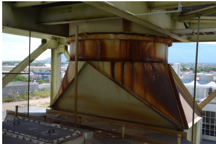
Figure 10 Unit 1 Stack Base
