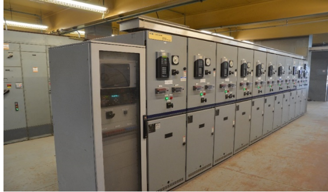
Figure 11 5 kV Switchgear
