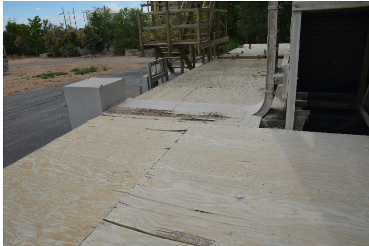
Figure 8 Unit 1 Cooling Tower Basin Deck
