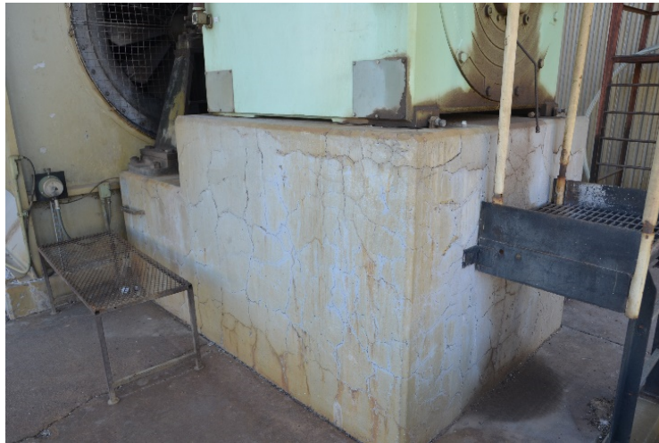
Figure 7 Unit 3 Forced Draft Fan Foundation
