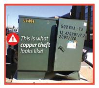
Once the copper is stolen, customers may find that even though their power is on, it fluctuates, electronics are sparking, or arcing is visible around the meter box or transformer. Copper thieves often leave open the transformers housed in the green metal boxes containing electrical equipment and live wires. **Touching them could be deadly. Stay away, never touch this equipment, and report it to PNM immediately by calling 888-DIAL PNM.**
