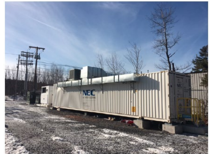
Sterling Municipal Light Department 2 MW, 3.9 MWh system
