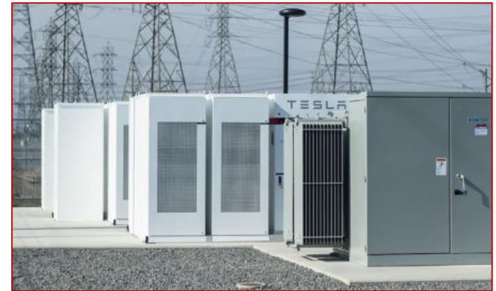
SCE/Tesla 20MW - 80MWh Mira Loma Battery Facility
