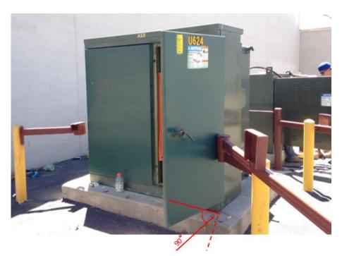
Transformer doors need to open <u>past</u> the 90° mark so that the door latch can lock, making it safe for linemen to work on the transformer
