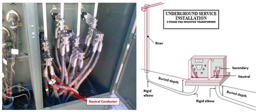
This is a single conduit, 4 wire 3φ power representation shown; with the fourth conductor (shown in white tape and connected to the HoXo lug) being the fourth wire. The neutral wire is designed to carry residual, unbalanced, or net current back and is the cable that is being stolen.
