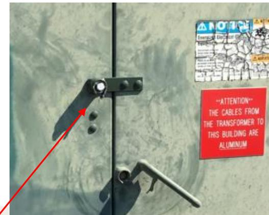
Retrofit door latch system for the transformer by PNM
