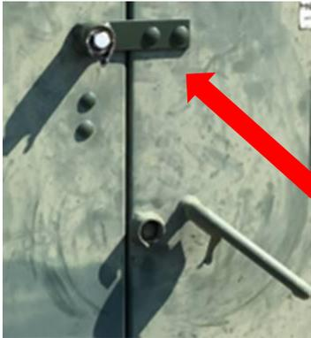
Existing transformer handle w/ pentahead as delivered by manufacturer
