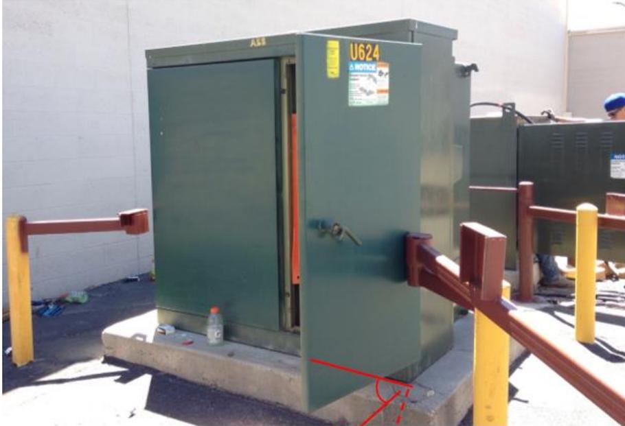
**Transformer doors need to open past the 90° mark so that the door latch can lock, making it safe for linemen to work on the transformer**
